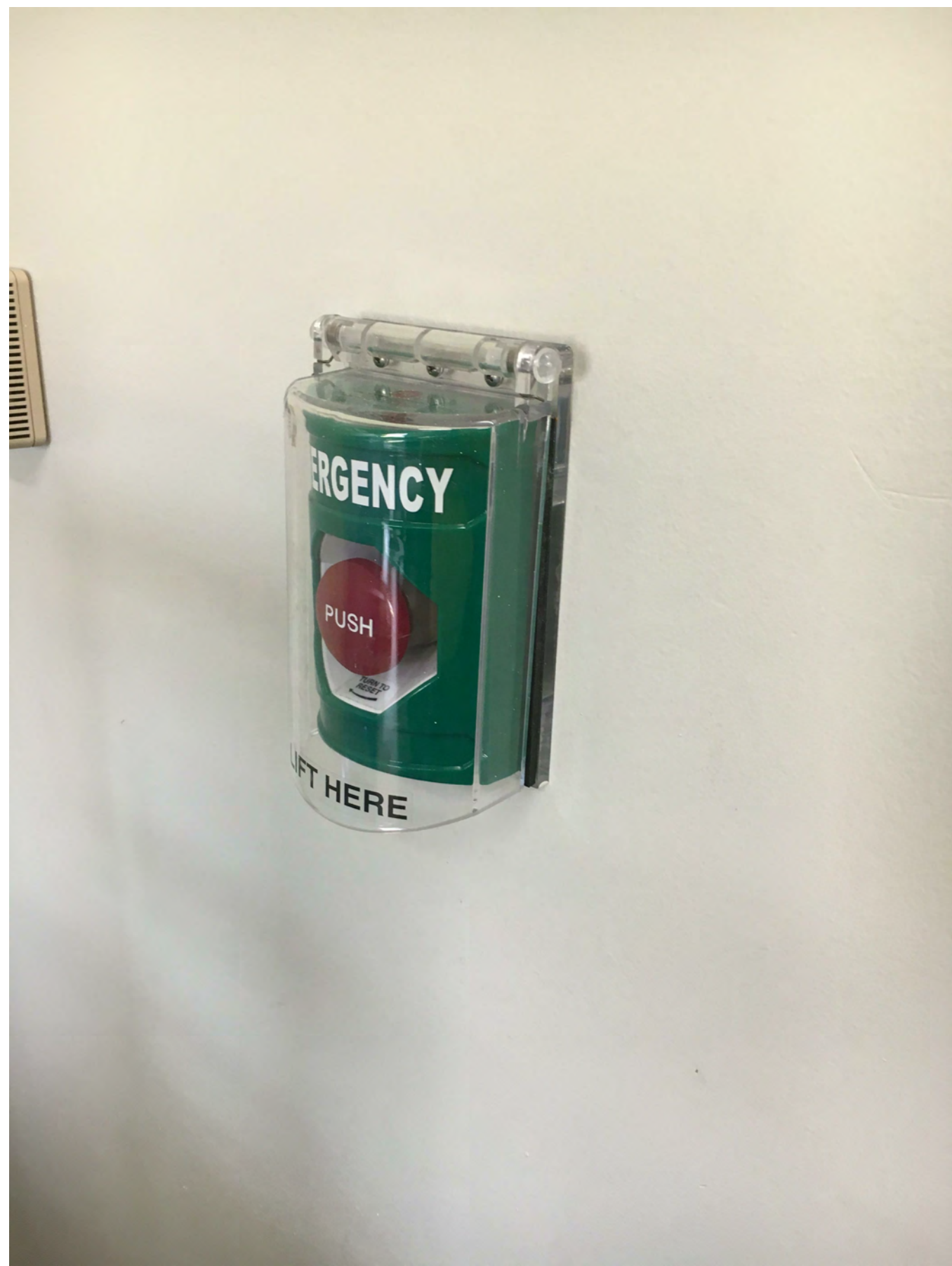
3 ED1.2E EMERGENCY DOOR RELEASE SCALE: NTS
