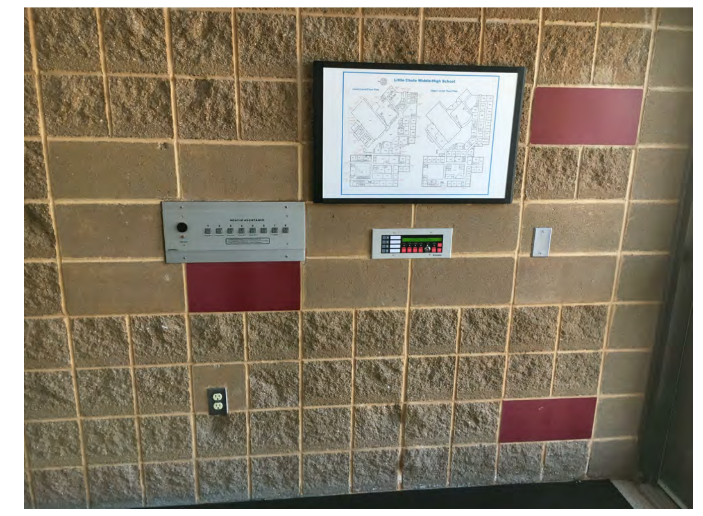
1 ED1.2B EXISTING AREA OF REFUGE MASTER AND FIRE ALARM ANNUNCIATOR SCALE: NTS
